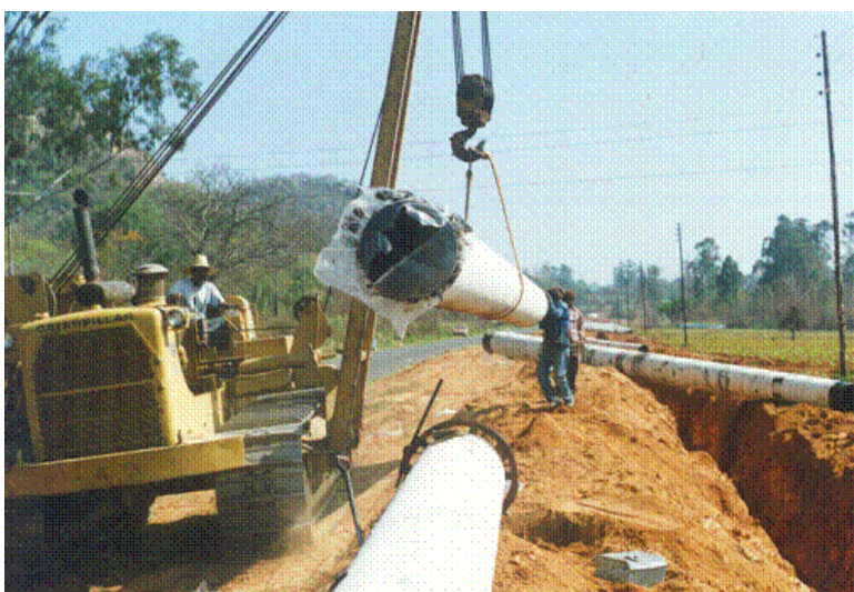
Figure 16: Trench and working area for pipe laying
